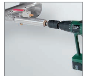
Drilling under pressure with CS drilling jig
